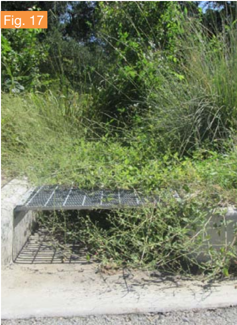
Curb inlet blocked by vegetation
