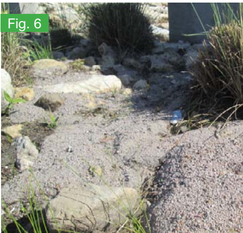
Sediment deposits that need to be removed
