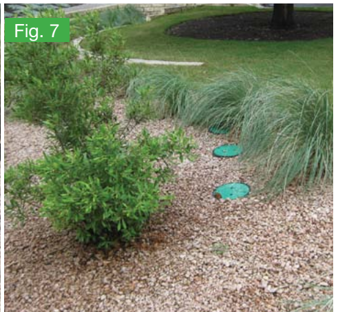
Bottom of the basin is clear of sediment buildup
