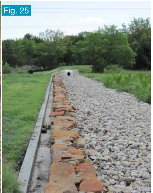
Unobstructed level spreader
