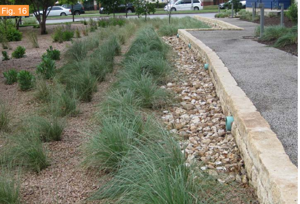
Inflow into the basin clear of all blockage
