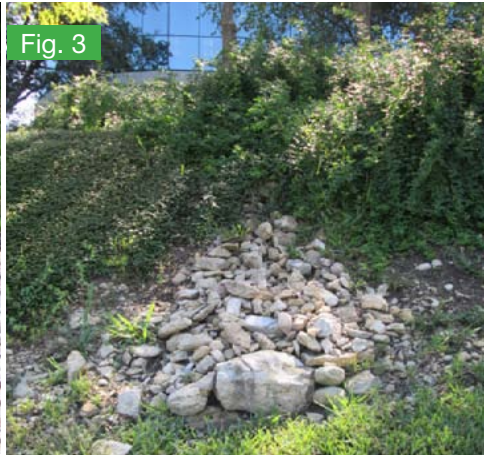
Scouring filled with 3-inch river rock
