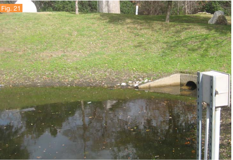
Holding water with no infiltration
