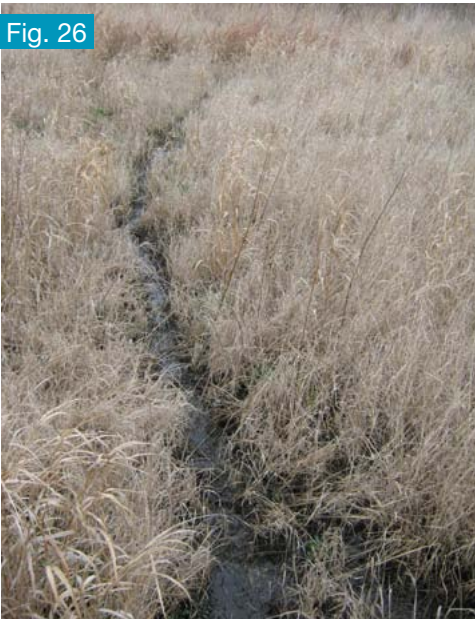
Vegetative Filter Strip showing rills caused by concentrated flow
