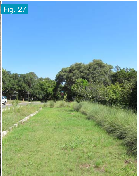
Vegetative Filter Strip with no rills or gullies
