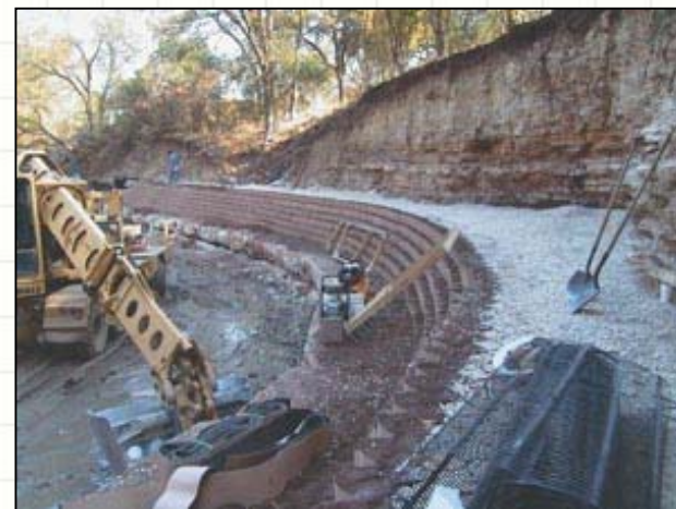
Erosion Repair: West Bouldin Creek
