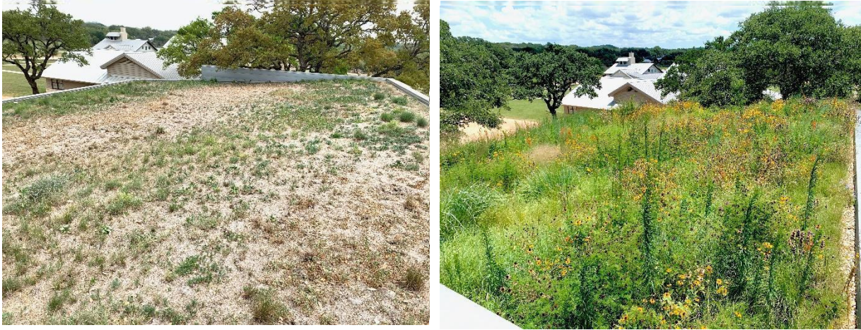
Figure 6-3. Native Prairie mix green roof in Wimberley Texas. The roof is growing in shallow media (6 inches) giving the community no access to water stored deeper in the soil column. Its position on a roof top exposes it to more extreme fluctuations in temperature than those on the ground (Simmons 2015). The image on the left shows the roof after being deprived of water for three months (April-June). The image on the right shows the community's recovery following the application of water.
